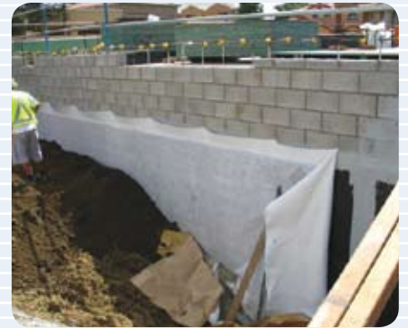
Wall panels for relief of hydrostatic pressure ensuring long term wall integrity.
