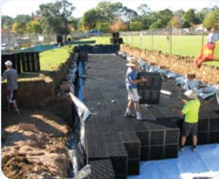
Underground tanks are ideal for rainwater harvesting for reuse and irrigation.
