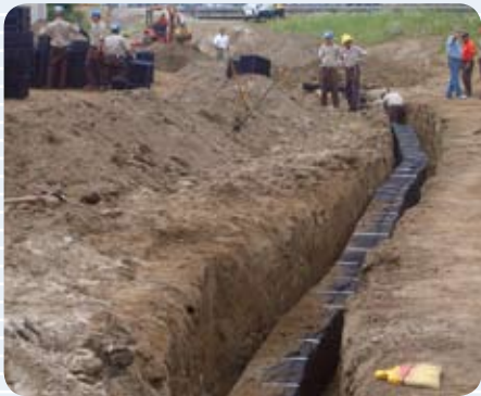
Channels to collect and infiltrate excess water.
