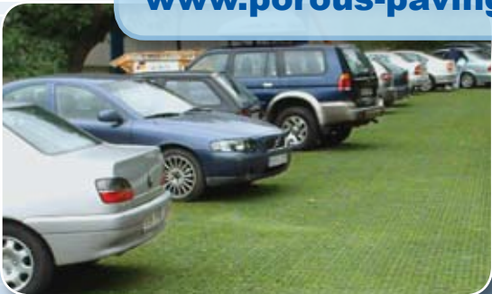
Turf Cell® installation for a parking lot
