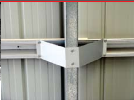
BRACING DETAIL
