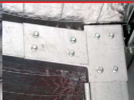
C FRAME EAVE CONNECTION
