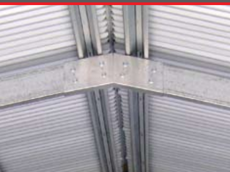
C FRAME RIDGE CONNECTION
