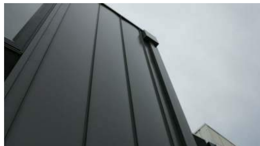
Metal wall cladding to be Lysaght "Longline" metal sheet cladding. Colour to be Colorbond "Monument"
