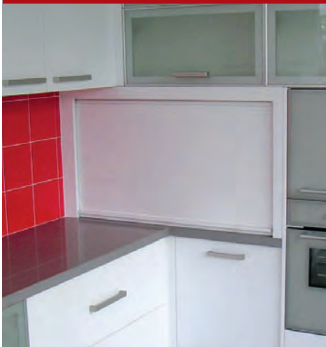
• Roller shutter in corner above bench top.
